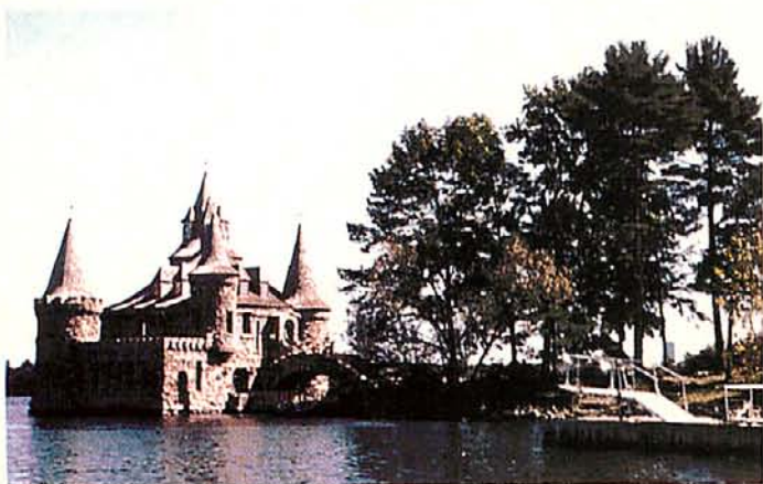
The power generator of Heart Island Castle is a miniature version of the main castle located nearby.
